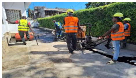
Engineers lay new tarmac for the compound
